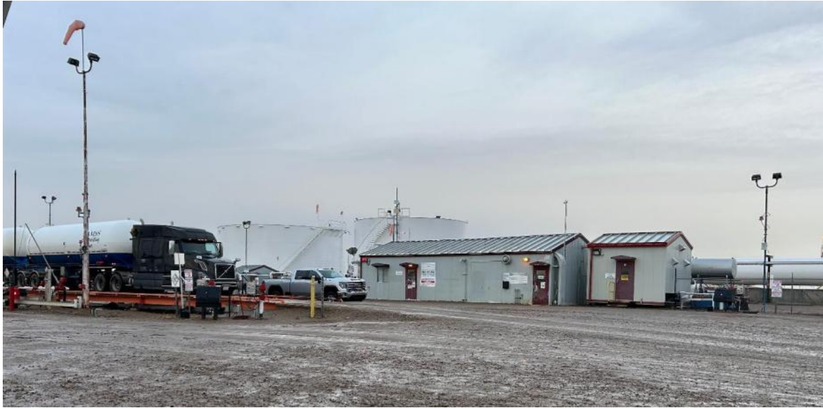
CER and Adjacent Facilities - Truck Scale, Tanks 104 (left) and 103 (right)
