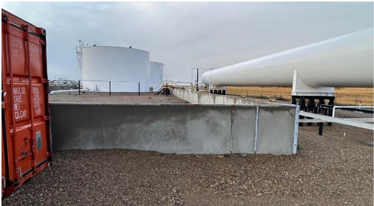
CER and Adjacent Facilities - Tank 103 & 104 in a Common Berm
